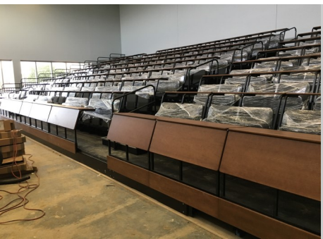
Recently installed Audience Systems Telescoping Lecture tables and seating, at South Louisiana Community College in Lafayette, LA.
